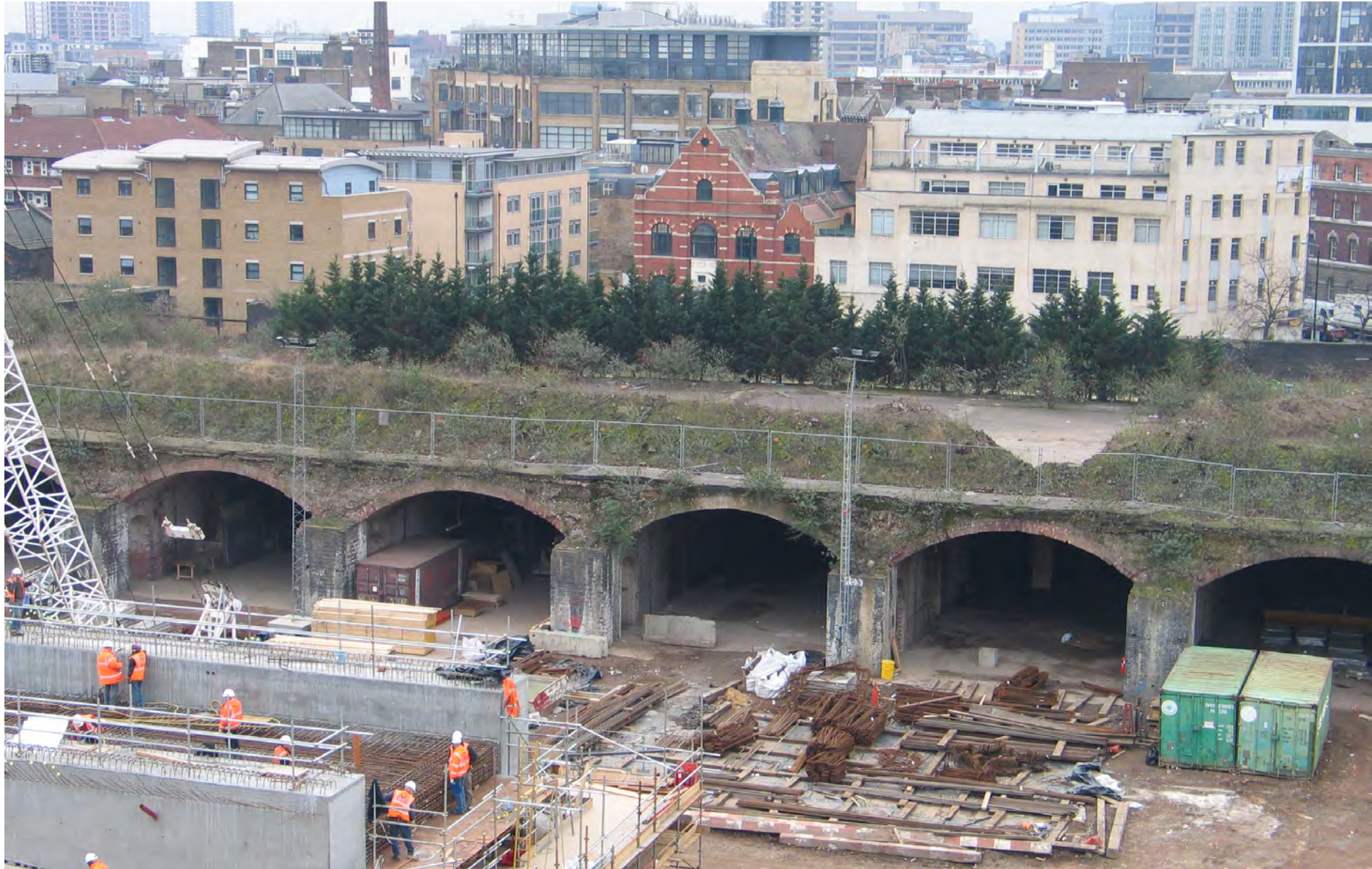
Fig. 31: Grade II listed Braithwaite Viaduct
