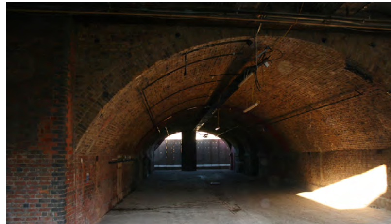
Fig. 30: Grade II listed : Arches beneath Braithwaite Viaduct
